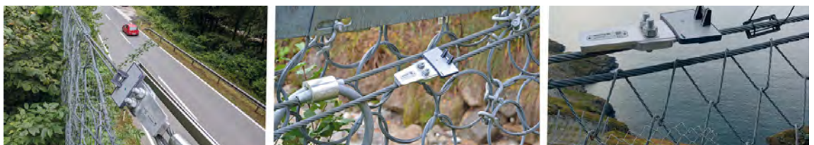
Fig. 2: Sensors on different components of rockfall barriers
