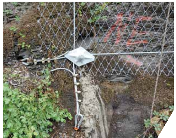
TECCO®-Slope Stabilisation (Anchorage of Border Rope)
