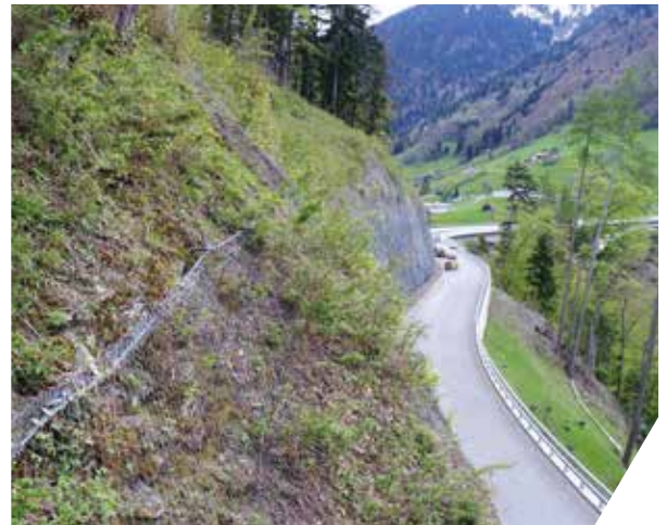
Rockfall Drapes (Anchorage of Support Rope)
