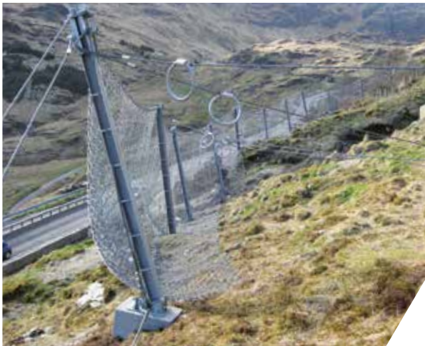
Shallow Landslide Barriers
