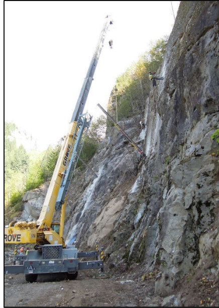
Figure 4. Construction of test Attenuator
