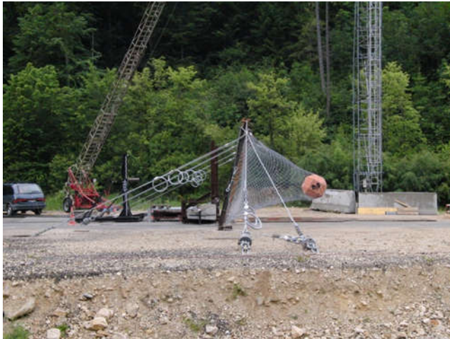
Figure 3. 500 kJ rockfall impact into a standard SL 150 shallow landslide barrier.
