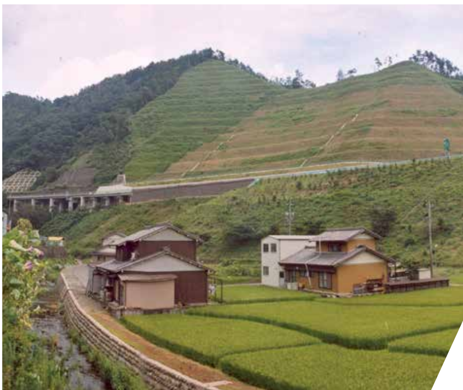
Fig. 6: Implemented project in Japan
