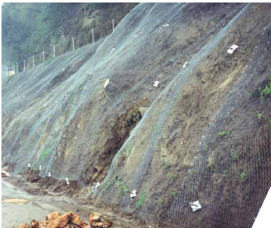
Fig. 40 (right): Protected slope in raw state
