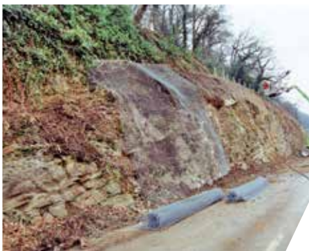
Fig. 39: Laying of the mesh sheets
