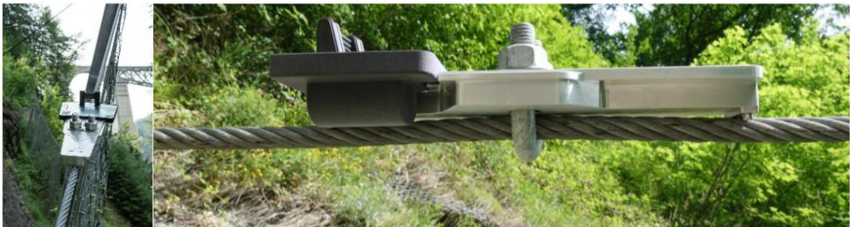
Figure 4: Correct installation of a Gebrugg GUARD device on a flexible protection system using a torque wrench. Integration of the GUARD into the platform (dashboard) using a mobile phone on-site.
