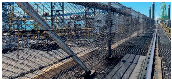
Geobrugg tailored protection solution at Hay Point
