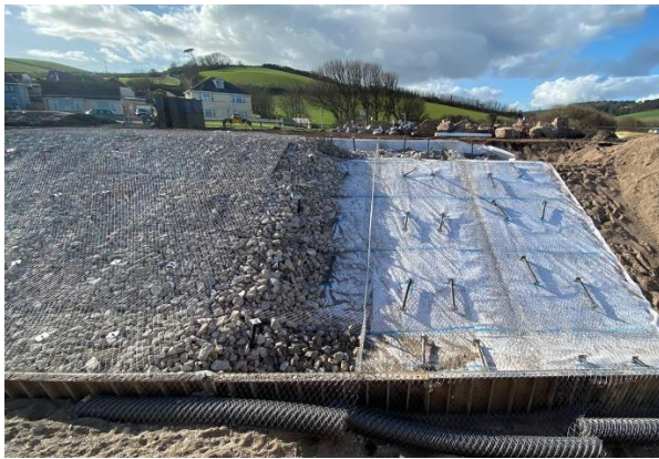
TECCO®Cell: installation in 2021 Picture: [E]
