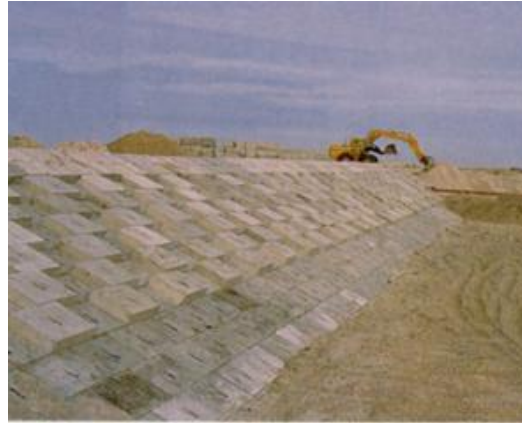
2. Precast concrete elements
