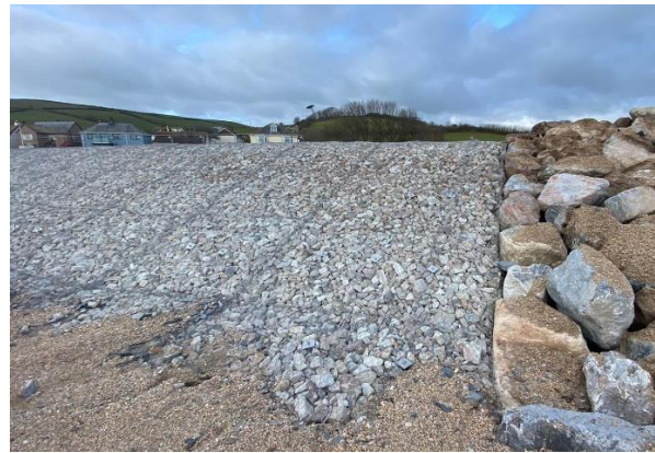
Finished installation of shore protection in 2021 Picture: [E]
