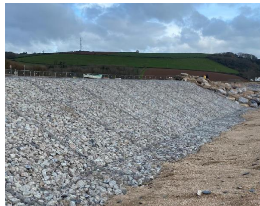
TECCO®Cell installed as shore protection Picture: [E]
