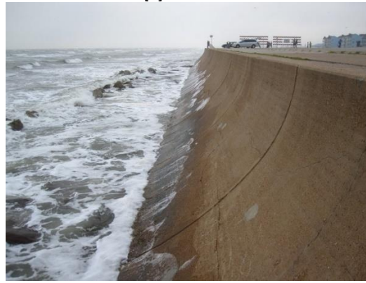
4. Curved concrete seawall
