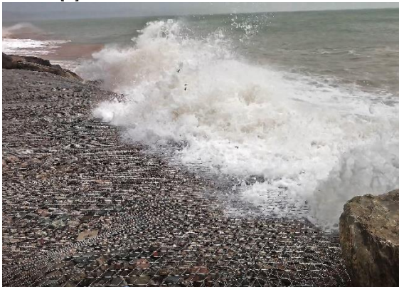
3. Steel mesh cells filled with blocks, stones and pebbles
