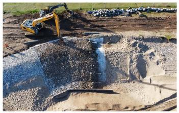
TECCO® CELL wrap design is constructed on site using custom designed bracing and connecting components and locally sourced fill materials of various grades. TECCO® stainless steel mesh which is quickly and efficiently constructed to form a 'cell' encasing fill
