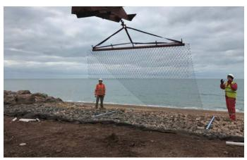
material and bracing/tensioning components. The system offers minimal impact on the landscape yet gives optimum protection to the interface between the beach and its surroundings.
