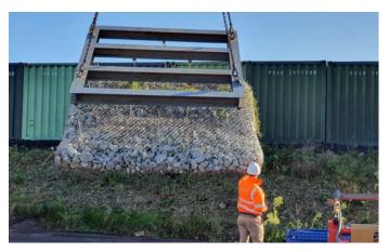
This solution is simply positioned as required in the problematic area with minimal preparation or excavation. Cells can be interconnected, however linking of the cells is not necessary as the substantial weight of a single cell provides stability and efficient protection against further erosion of a small area to the local environment.
