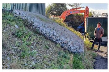
Eroded coastal sections that are not directly connected to traffic routes are the rule rather than the exception and often worthy of protection. In these circumstances TECCO® CELL Mobile can be deployed quickly to stabilize the location with a minimum of disruption to the local environment.
