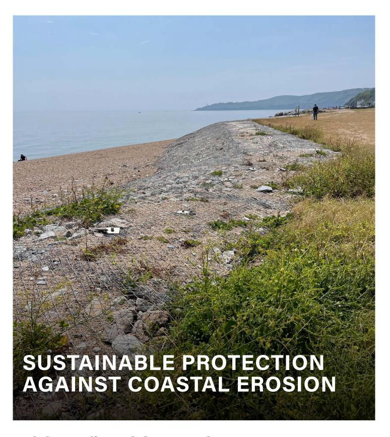
High-tensile stainless-steel wire mesh system
