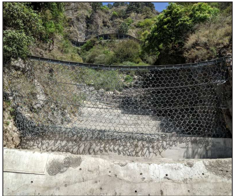
Installation of Debris Flow Barrier at Location no.-32 &33
