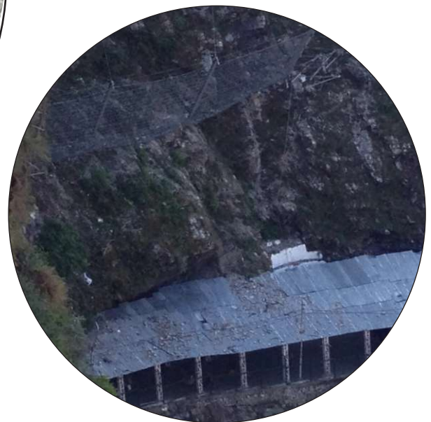
View of Installed Rockfall Barriers at Location no.-16
