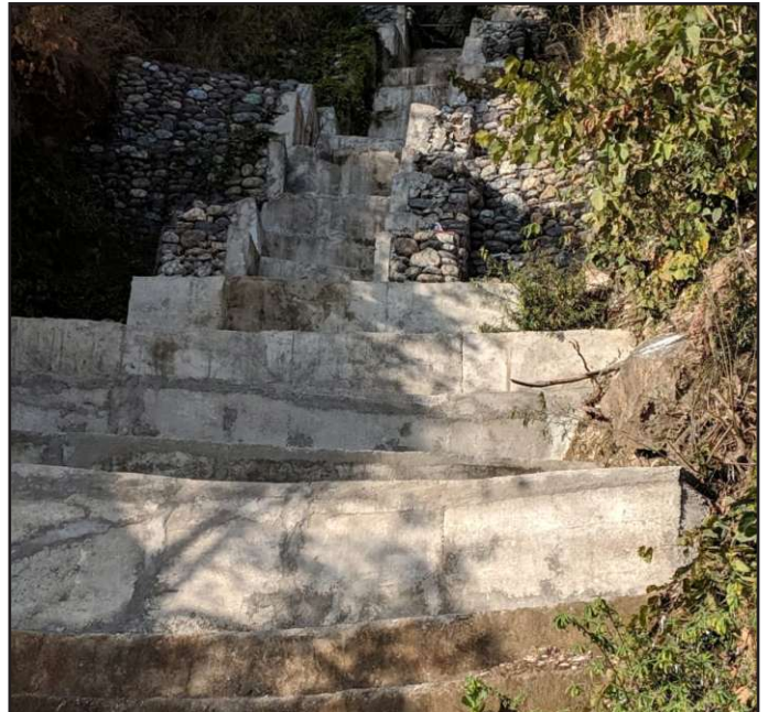
View of gabion channel at Location no.-32 &33
