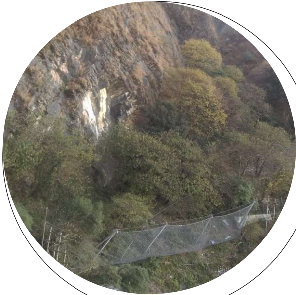
View of Installed Rockfall Barriers, Location no.-17
