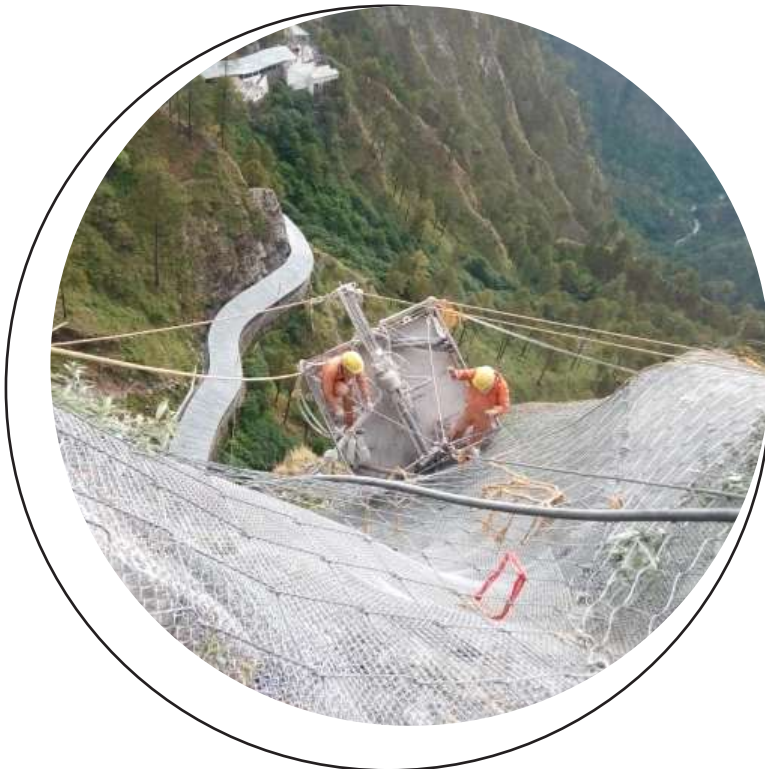
View of High Tensile Steel Rolled Cable Net at Location no.-14
