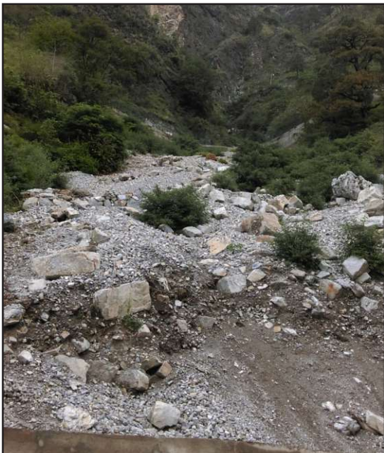
View of debris flow crossing nalas at Location no.- 32 &33
