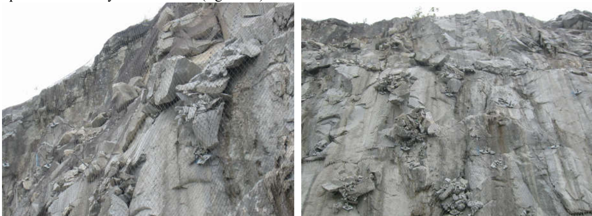
Figure 16. Tecco® stabilization system containing large blocks
