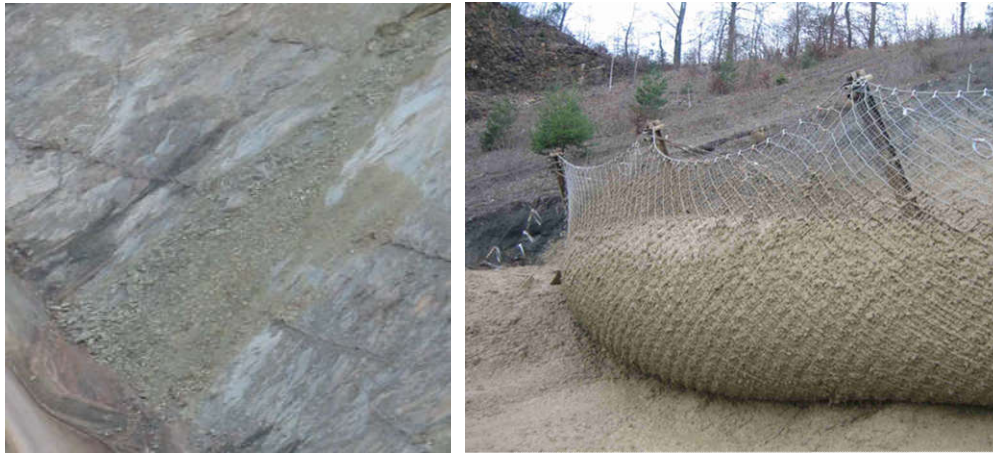
Figure 9. These catch fences are not adequate to stop a small rockslide (left) and shallow landslide barrier during test.
