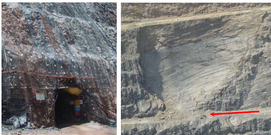
Figure 8. Portal to underground operation (left) and failure in a pit wall (right).
