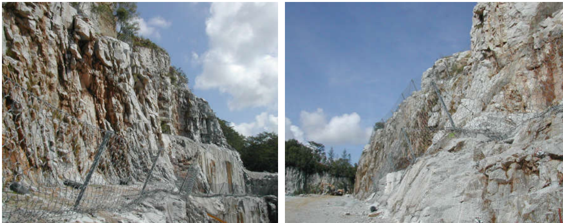
Figure 15. Lateral and bottom view of the barriers once installed
