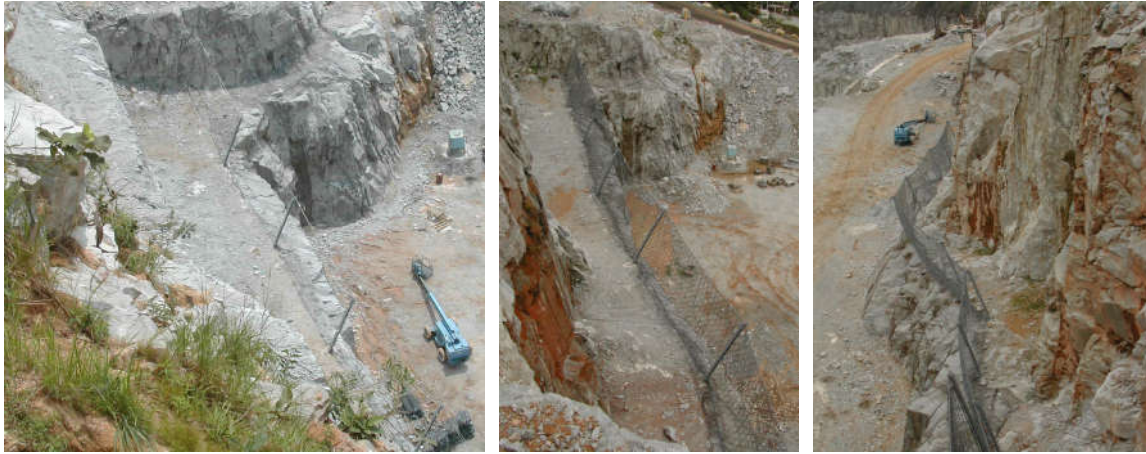
Figure 14. Top view of the barriers during installation
