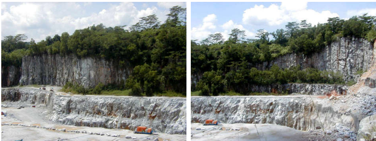
Figure 11. Chainage 360 – 560 (left) Chainage 540 – 640 (right)
