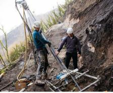
Simple installation In the case of loose subsoil, self-drilling anchors are particularly advantageous. The FLEX Head is simply screwed onto the anchor, then the concrete foundation can be prepared around the anchor.
