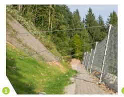
**Low anchor forces - high efficiency** The innovative construction allows the rockfall energy to be dissipated particularly by the ring net panels and the brakes.
