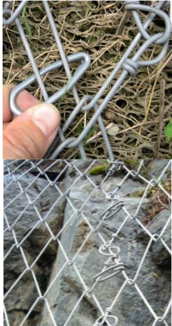
Figure 3. T3 Clip used to connect TECCO panels vertically in rock (lower) and in soil application (upper).
