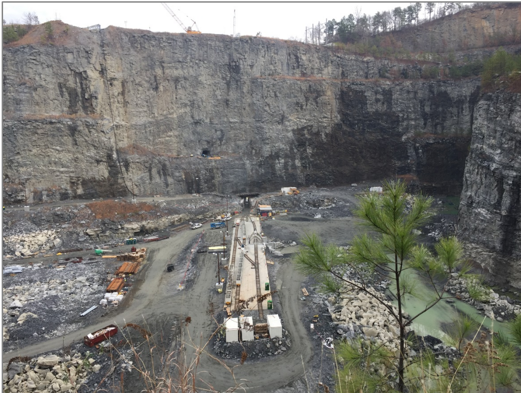
Figure 1 – Northerly view of quarry highwall, tunnel and adit (on bench) (Photo by Scarptec, Inc.)
