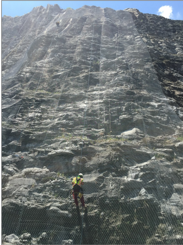
Figure 2 – Constructed rockfall drape (Photo by Scarptec, Inc.)
