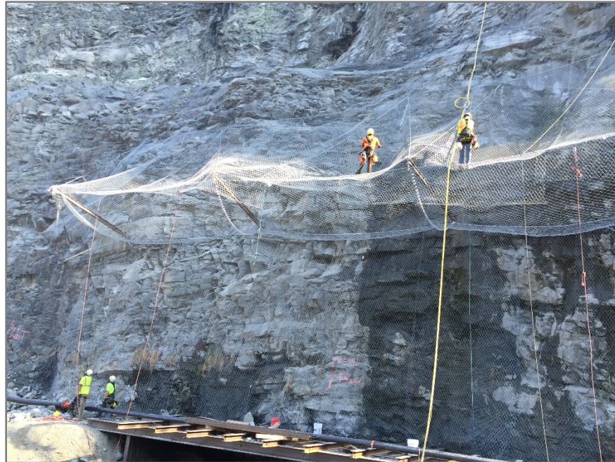
Figure 5 – Canopy construction and drape tie-in (Photo by Scarptec, Inc.)
