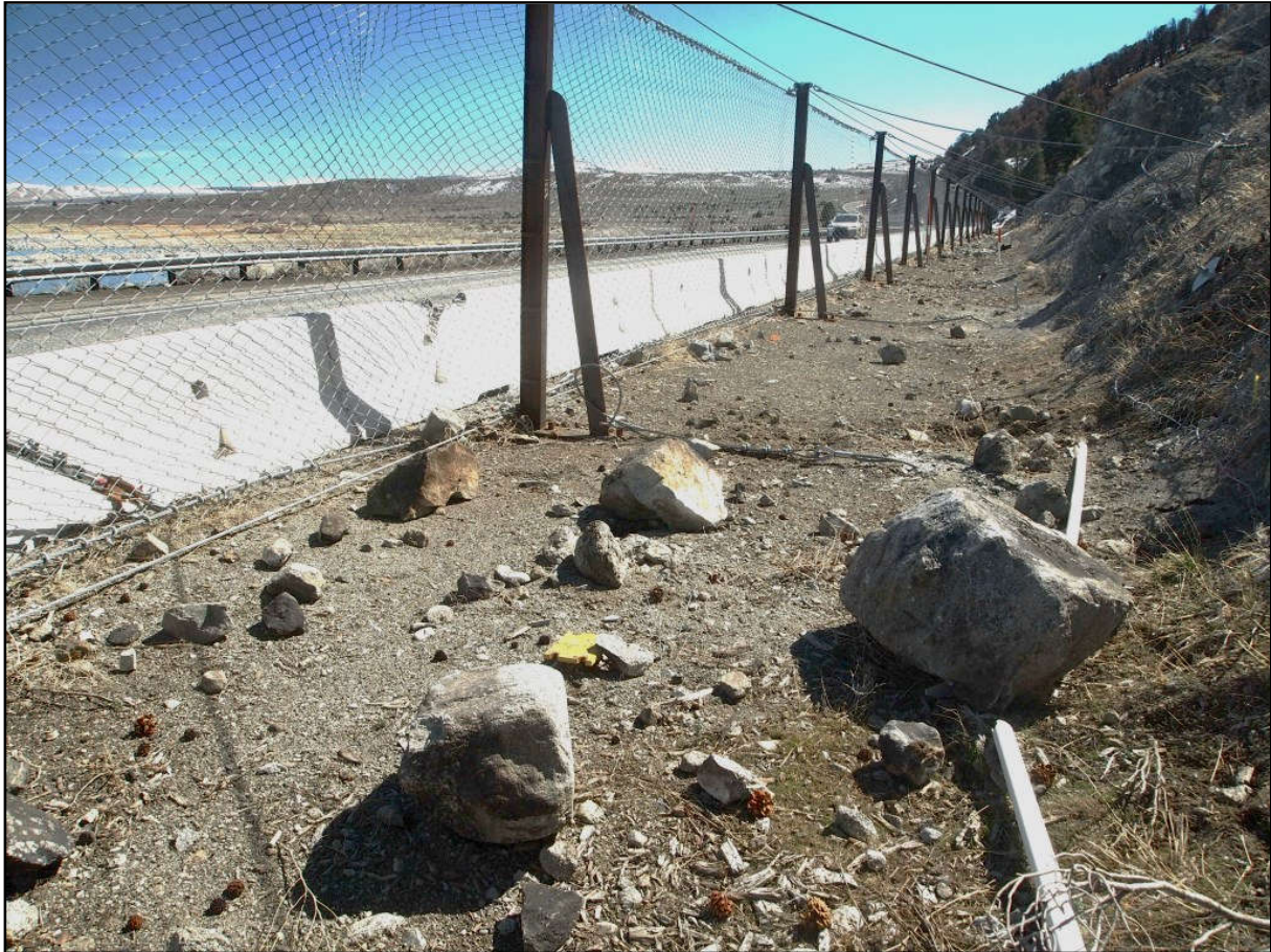
Figure 8. Rockfall event occurring on March 12, 2017 retained behind 3m Geobruigg GBE500AR flexible rockfall fence. (Photo credit: Joe Blommer, Caltrans)
