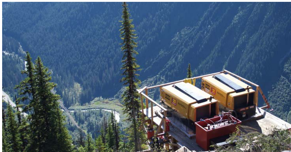
One of three equipment pads
