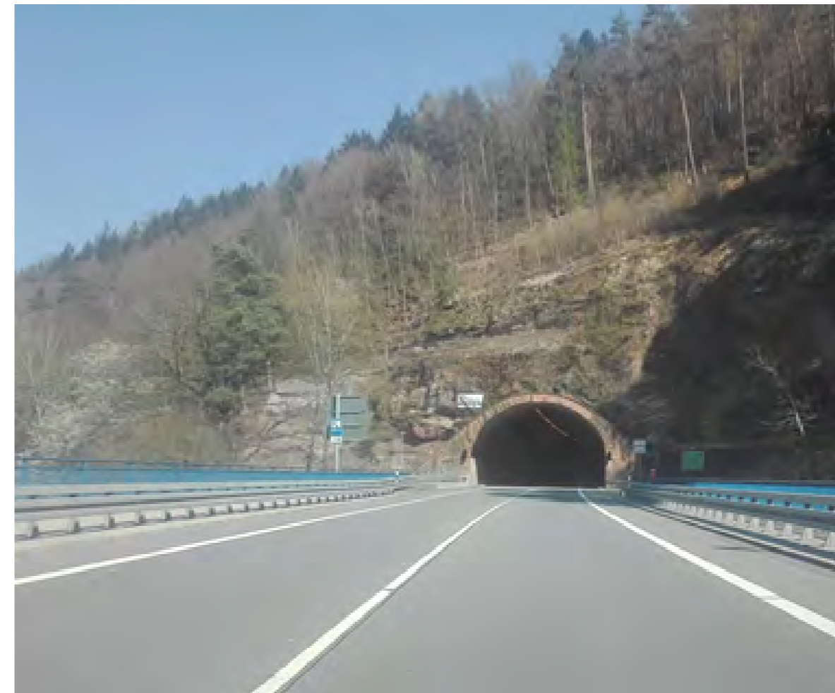
Entrance of the Hirschhorn Tunnel
