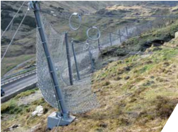
Shallow Landslide Barriers
