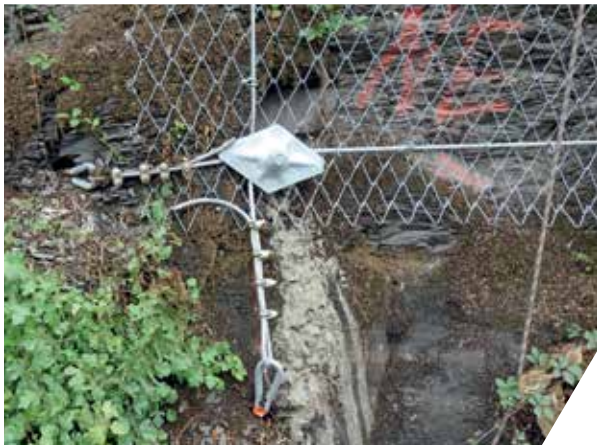
TECCO®-Slope Stabilisation (Anchorage of Border Rope)
