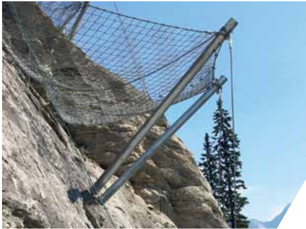
Avalanche Prevention with Spiral Rope Nets
