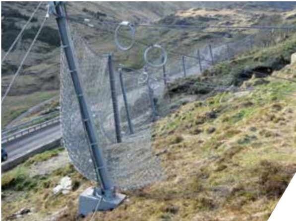
Shallow Landslide Barriers
