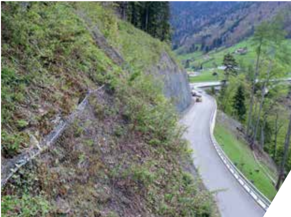
Rockfall Drapes (Anchorage of Support Rope)
