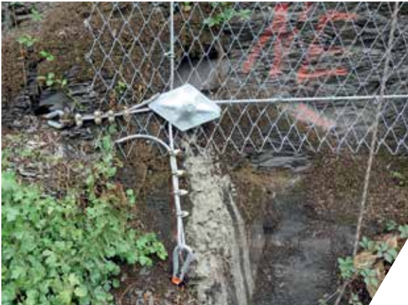
TECCO®-Slope Stabilisation (Anchorage of Border Rope)
