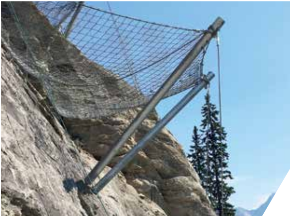
Avalanche Prevention with Spiral Rope Nets
