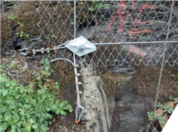
**TECCO®-Slope Stabilisation (Anchorage of Border Rope)**
