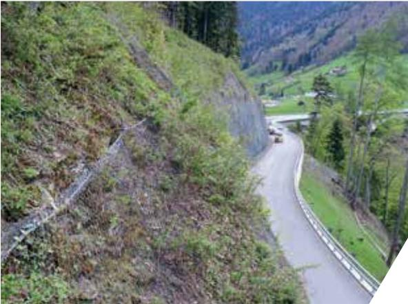
**Rockfall Drapes (Anchorage of Support Rope)**
