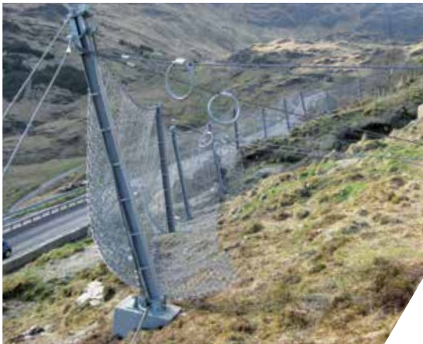
Shallow Landslide Barriers
