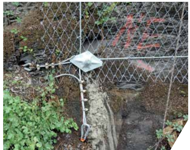
TECCO®-Slope Stabilisation (Anchorage of Border Rope)
