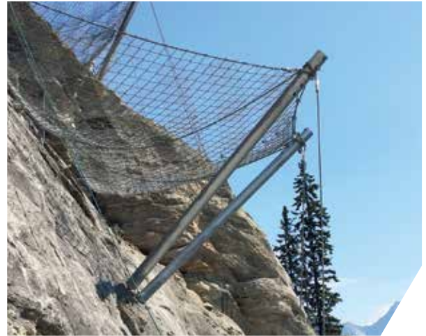
Avalanche Prevention with Spiral Rope Nets
