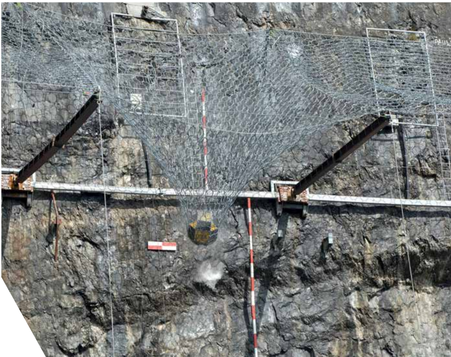
System in 1:1 field test: A test block falls into the netting before it is successfully redirected to a safe zone
