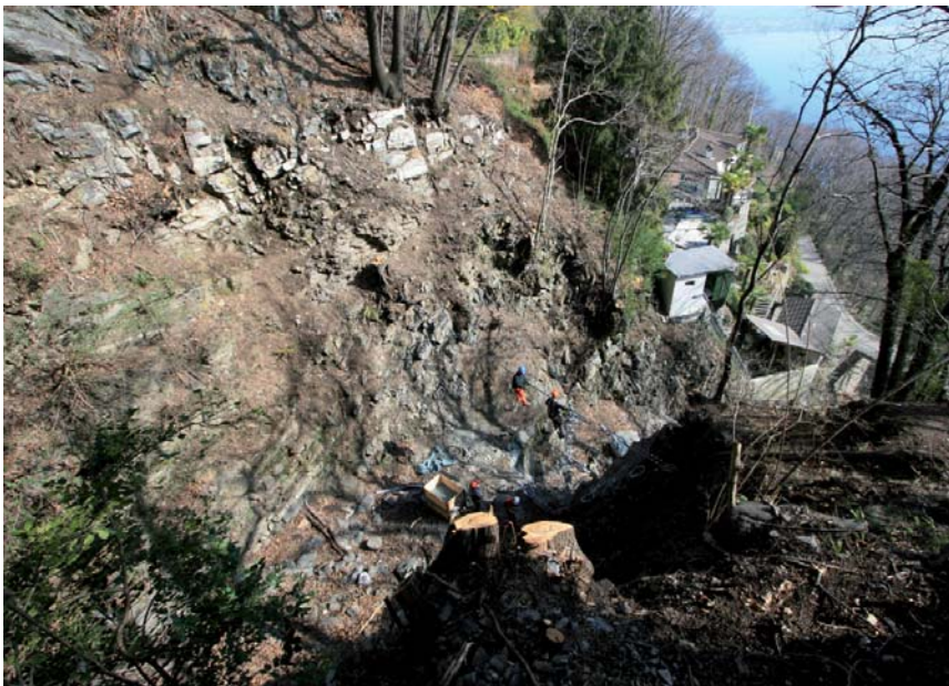
Fig. 2: View from above the area involving the works
