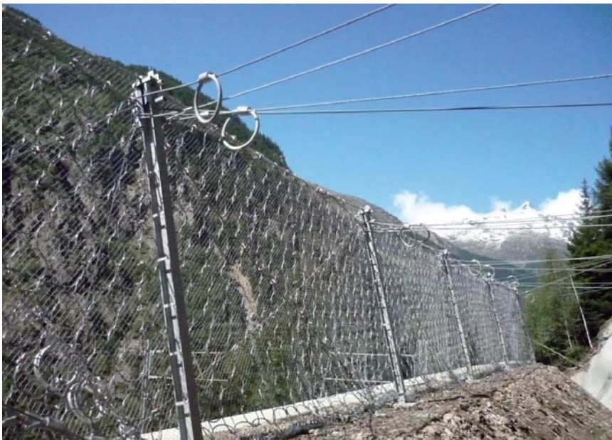
RXI-100 rockfall protection barrier with ring net and secondary mesh.
