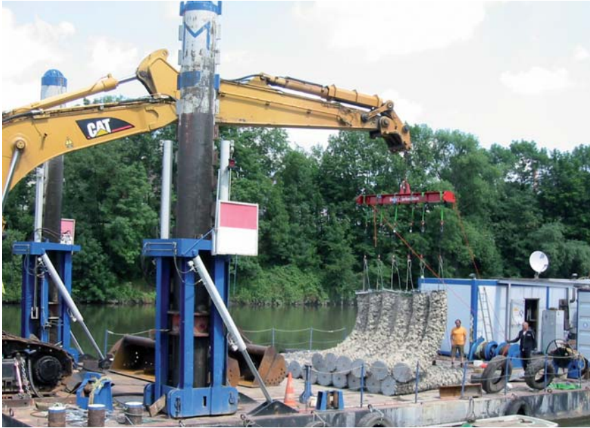
Unloading the TECCO® pillars
