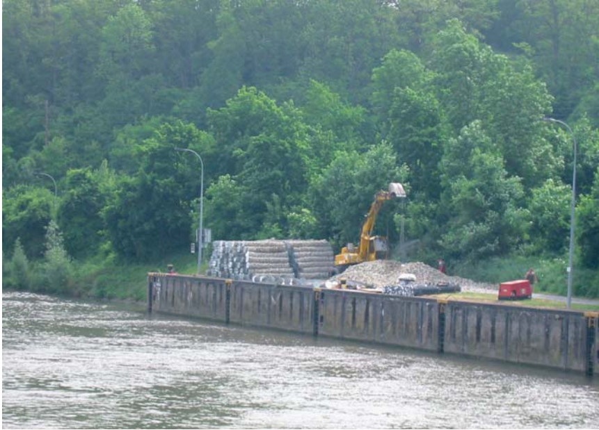
Empty pillar baskets prior to filling
