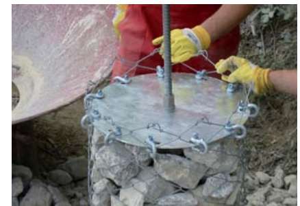
Pillar filling in vertical shaft, sealed by a cover with connecting bearing
