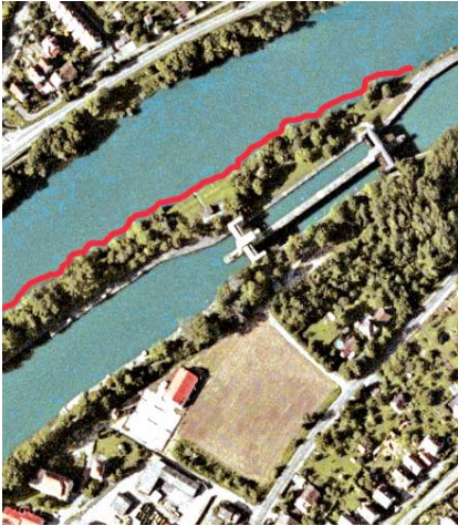
Aerial photo of the dam (extract from Google map; red line = construction zone)
