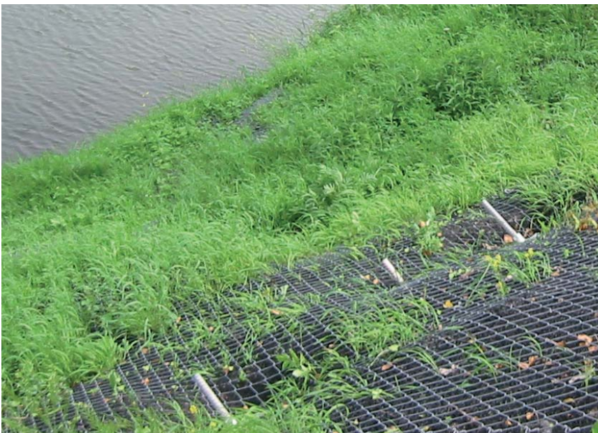
Fully stabilized dam
