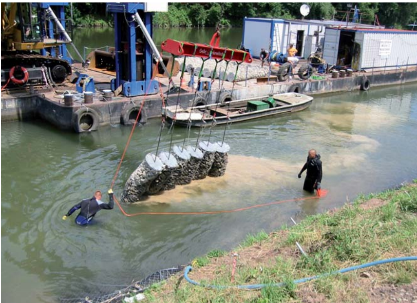
Divers assisting with the pillar placing
