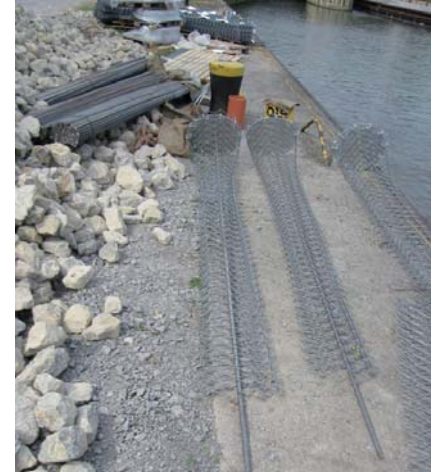
Empty pillar baskets prior to filling
