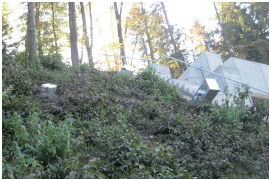
Overall view of the ABOXX installation
