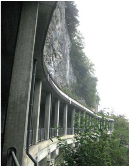
Rockfall protection gallery Mattstock and Churfiristen
