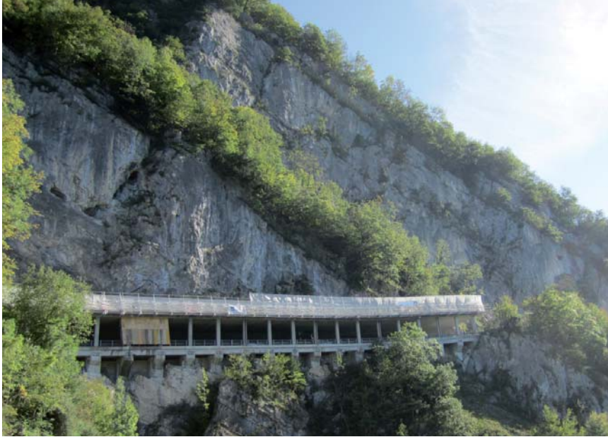
Possible breakout zone above the rock-fall gallery protection
