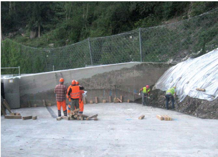
Excavated gallery roof and renewal of the joint sealings
