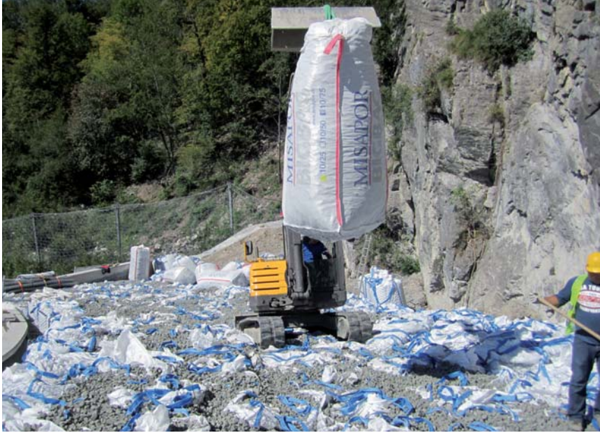
Filling of the gaps with cellular glass fill material
