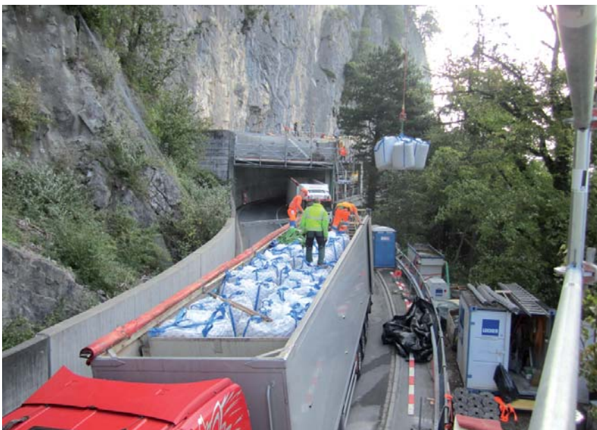
Delivery of the ROCKFALL-X™ damping moduls by truck
