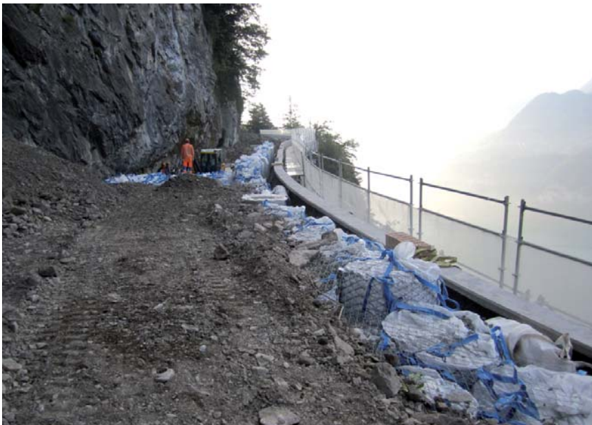
Regular gravel is placed above the installed ROCKFALL-X™ damping systems
