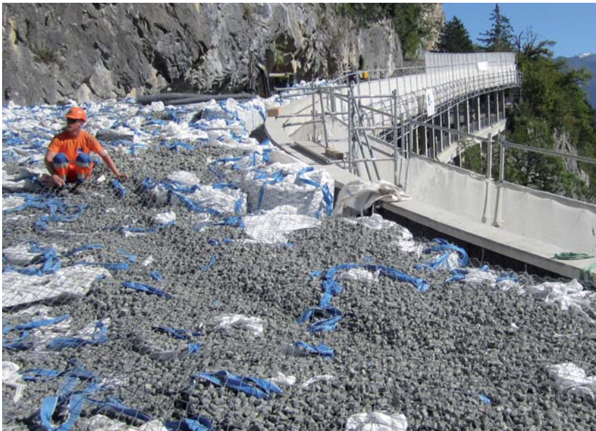
Installation of the TECCO® G65/3 horizontal mesh covering the damping system
