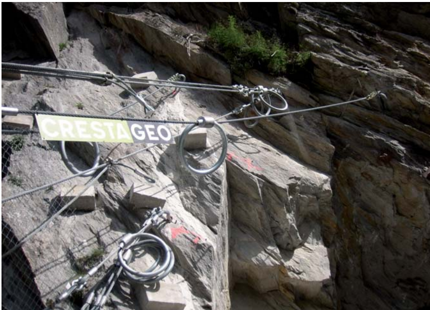
Lateral guy ropes with 6 m-long rope anchors.
